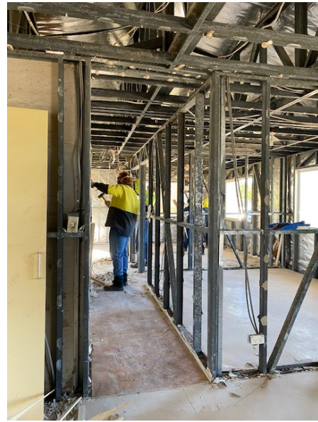
Some demolition photos of 33 Byrne Street
