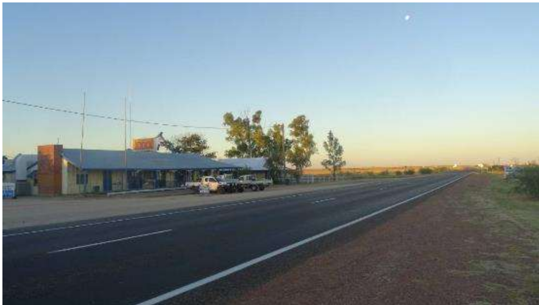
The Blue Heeler Hotel & Pub and Hulbert Street/Landsborough Hwy
