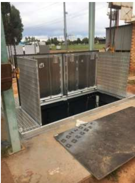
Safety Lid installation, displayed in its open form
