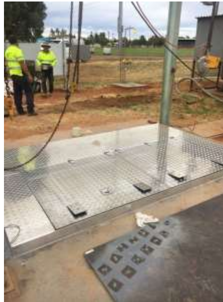
Typical safety Pump Well lid installation.
