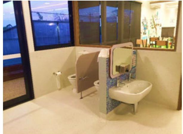
Toilets and handbasins. Note the handbasin which accommodates two taps
