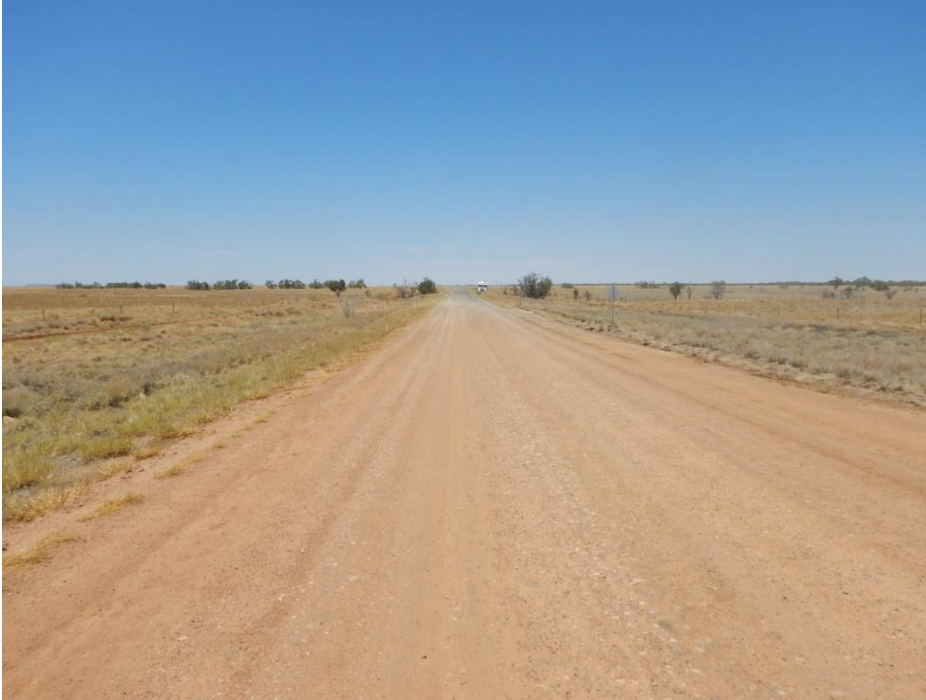
Cannington Road – Stabilisation – Prior to Seal
