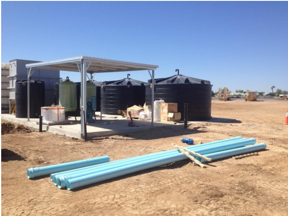
Julia Sewage Treatment Plant under construction
