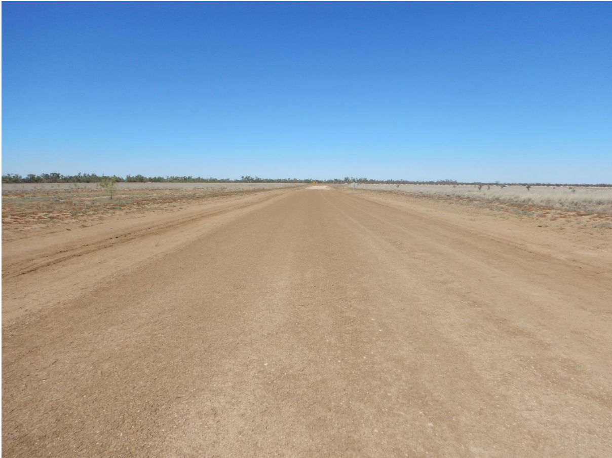
Punchbowl Road - Grading
