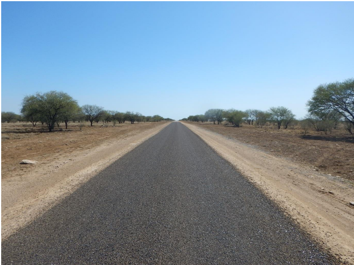
Punchbowl Road - Stabilisation
