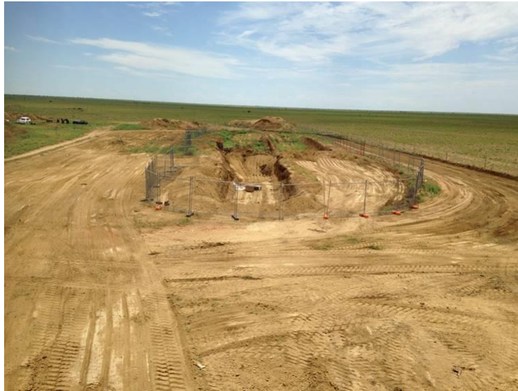
Picture 2 – McKinlay General Waste Pit after clean up
