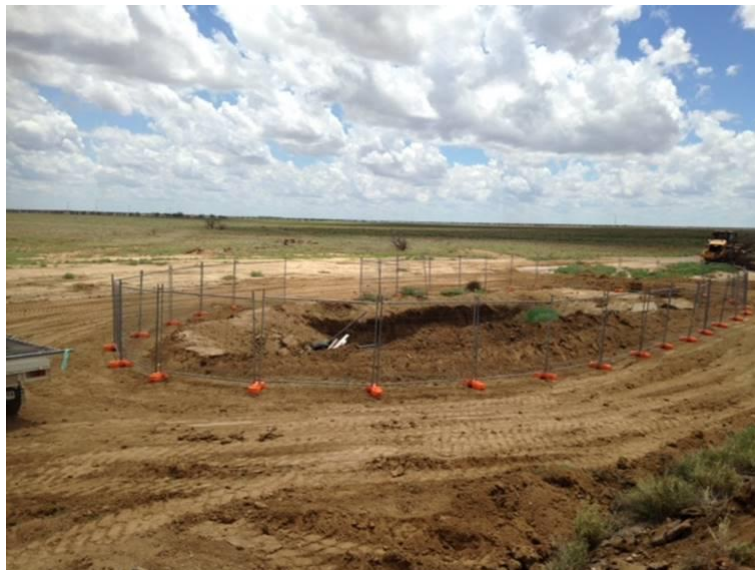
Picture 3 – Nelia General Waste Pit after clean up
