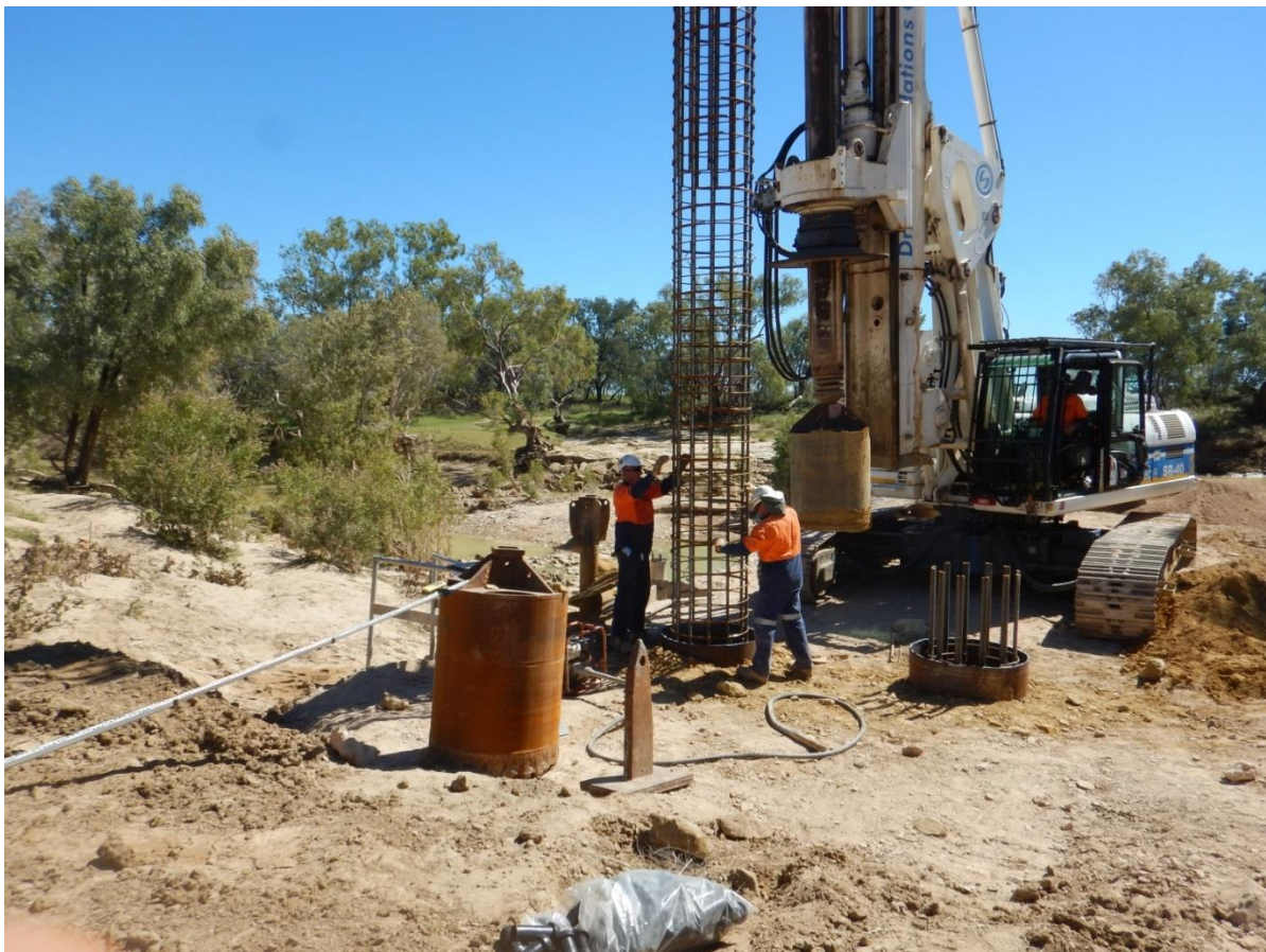
Figure 1 Punchbowl Bridge - Boring for Piers and Placing Reinforcement Cages
