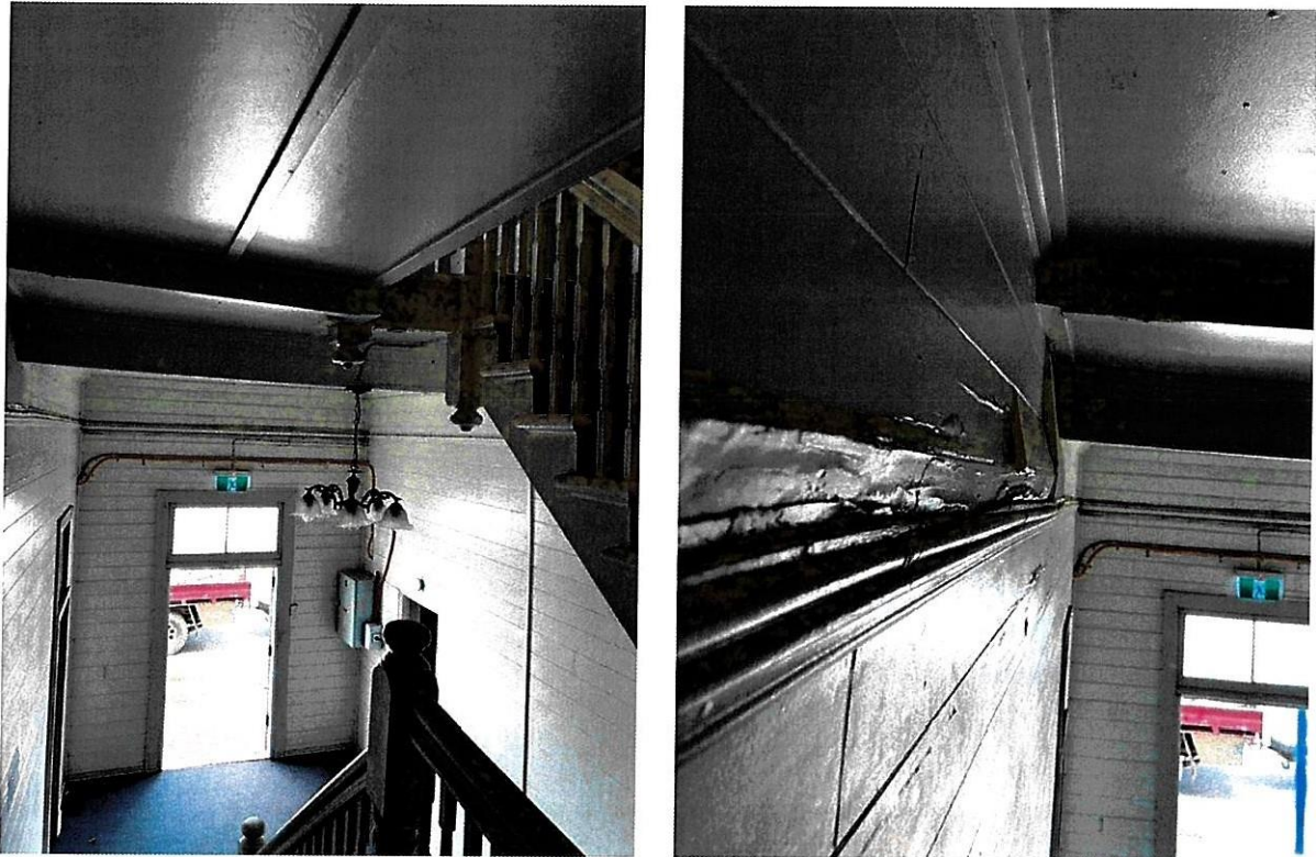
Figure 4-8 Condition of the Internal Stairs
