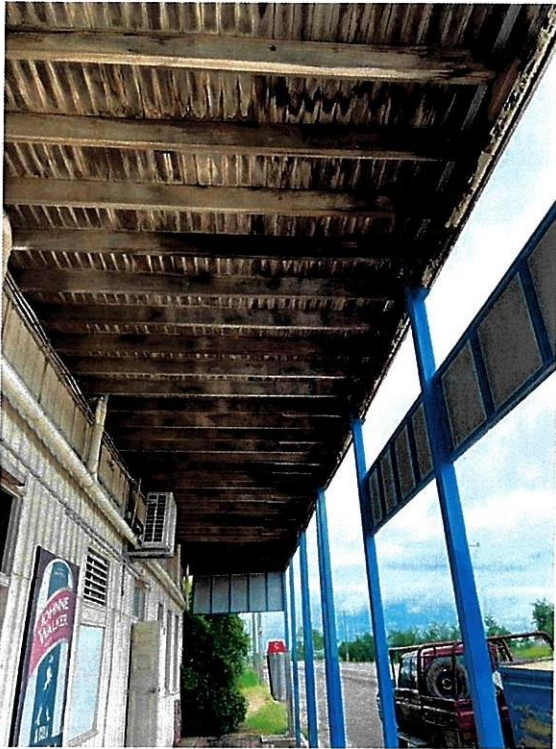
Figure 4-16 View of the South side of the front deck, with split bearer and deteriorated timber elements
