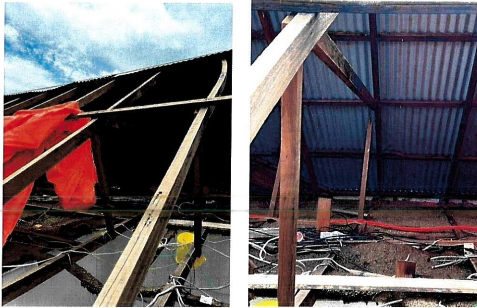
Figure 3-4 Current configuration and condition of the roof structure
