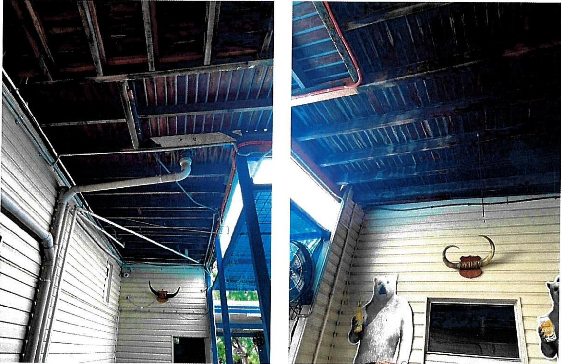
Figure 4-20 View of the rear deck from below
