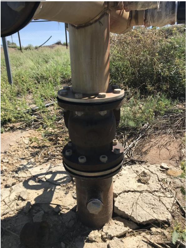
The scour bore head is in good condition. This bore was logged in November 2021. Minor cracks to the concrete around the base that requires removal and laying of new concrete to provide a stability platform around the pipe. This is outlined in the Risk Management Improvement Program in Section 6.1 of this plan.
