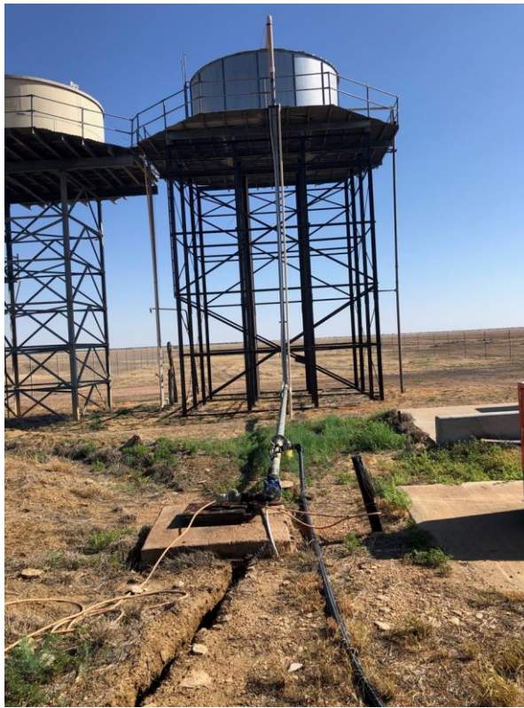
Figure 2.5 – Photo of the McKinlay Water Facility
