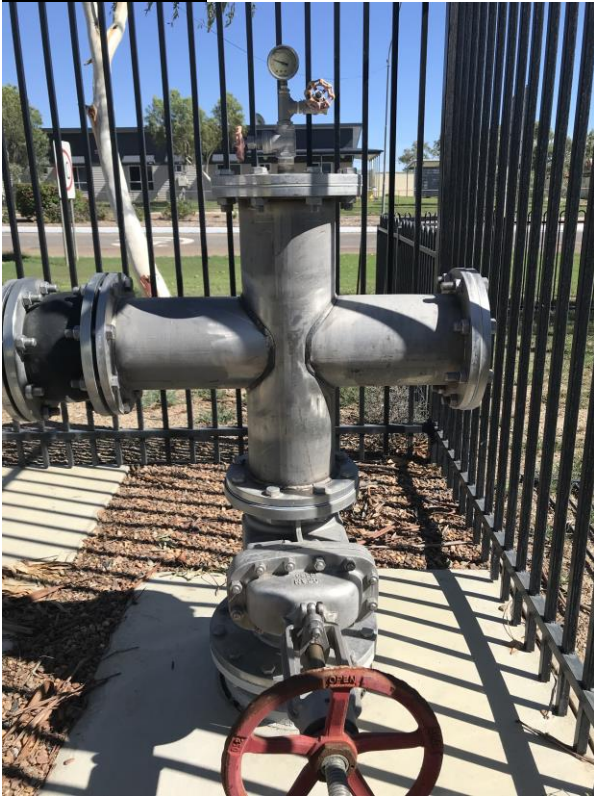
The lions bore head is in good condition. This bore was drilled in 2020.
