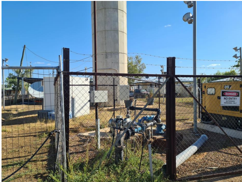
Figure 2 – Photo of Water Tower Bore
