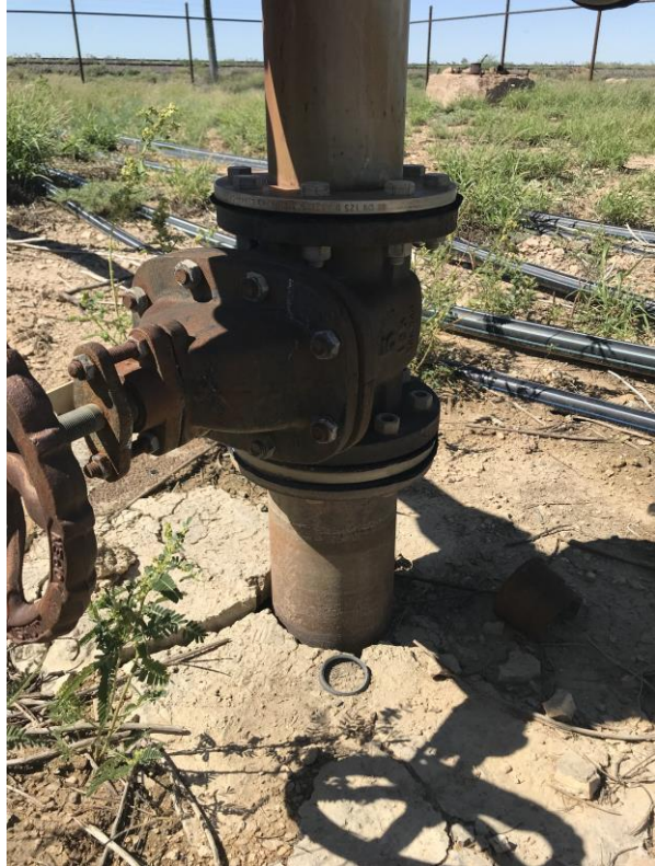
The scour bore head is in good condition. This bore was logged in November 2021. Minor cracks to the concrete around the base that requires removal and laying of new concrete to provide a stability platform around the pipe. This is outlined in the Risk Management Improvement Program in Section 6.1 of this plan.
