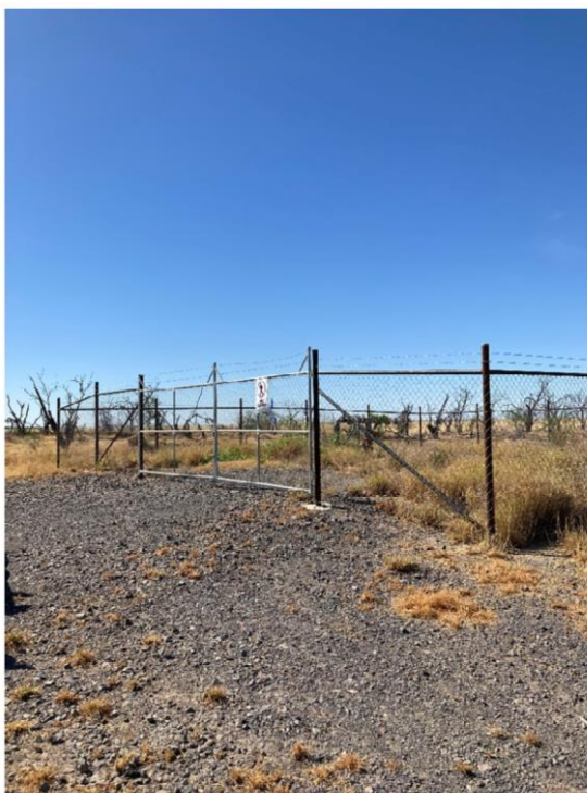
Figure 2.7 - Photo of Nelia Water Facility
