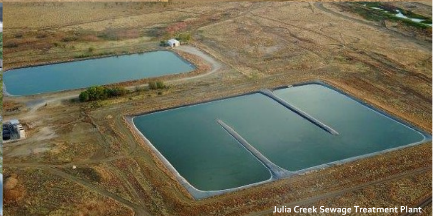
Julia Creek Sewage Treatment Plant
