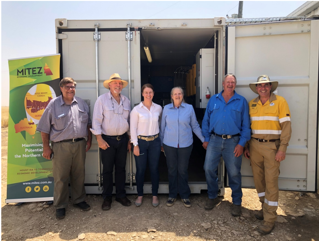
MITEZ, McKinlay Shire Mayor, Site Managers, and Ergon Energy visit the Power Pod on site after officially being connected on 17 October 2019.
