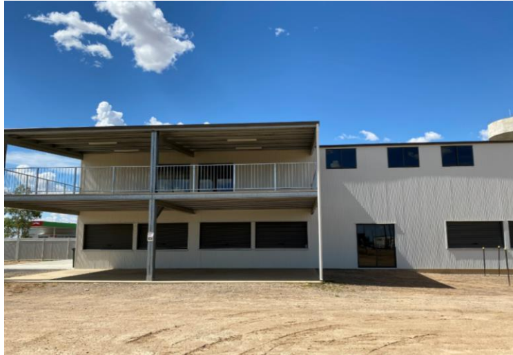
Figure 2: Dirt and Dust Building
